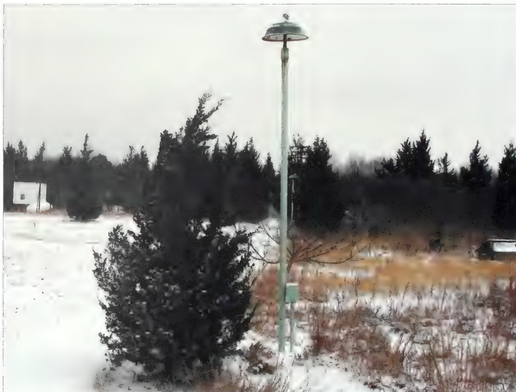
Figure 5.110. Existing light fixture, NIKE radar site. The historic light fixtures should be periodically inspected, have components repaired or replaced as needed, and receive corrosion treatment, priming, and painting to match the historic finish. The eastern red cedar in the foreground should be removed as part of vegetation management along the circulation systems (Olmsted Center, January 2009).
